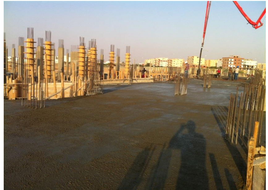
Pump for the concrete slab
