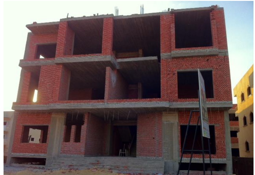
Completion of masonry work
