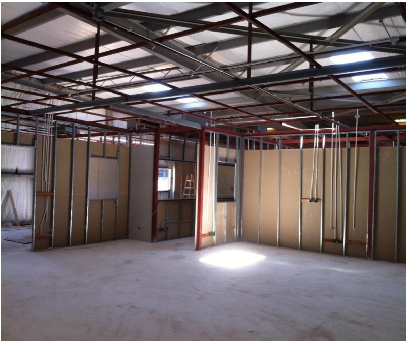
Electric works and gypsum partitions
