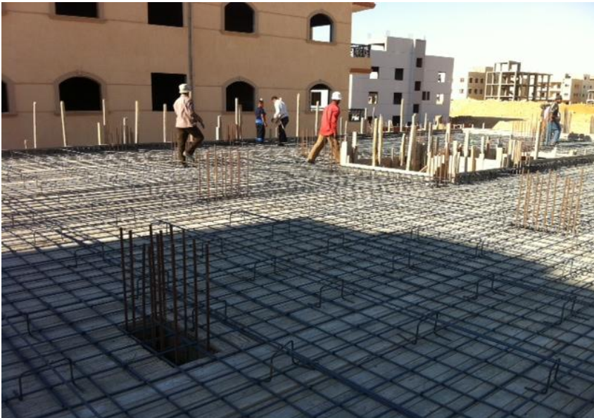
Steel Fixing of 1 st Floor slab
