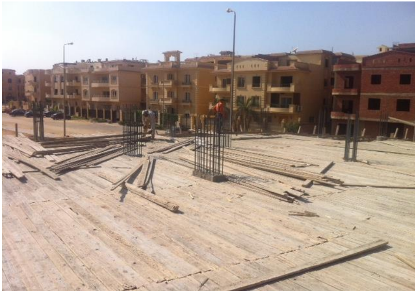
Formwork of Ground Floor slab
